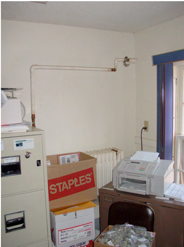
PR-2b: Office on south side of corridor with typical crowding.
