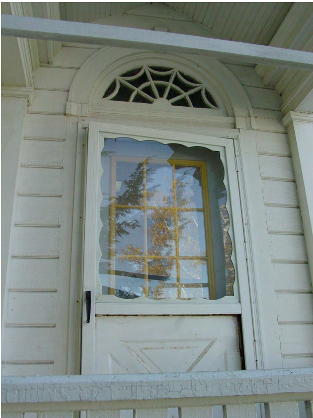
AI-2: Replacement door, exterior view.
