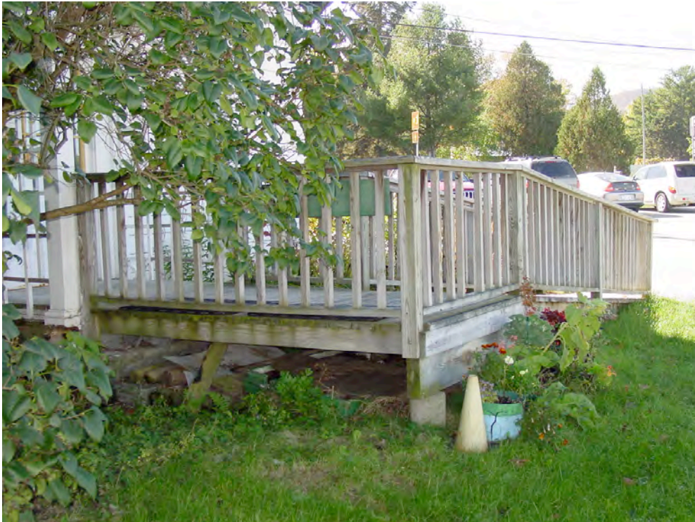
PR-5a: Existing ramp at northwest entrance.
