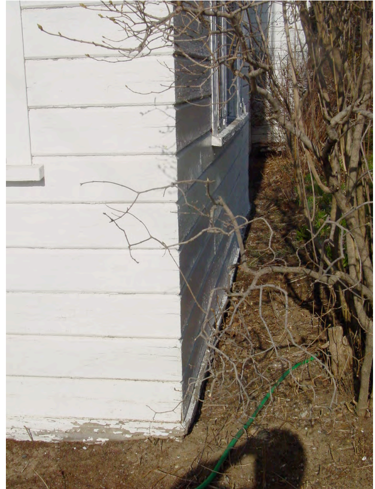
EC-4a: Detail of southwest corner with ground again wooden façade.
