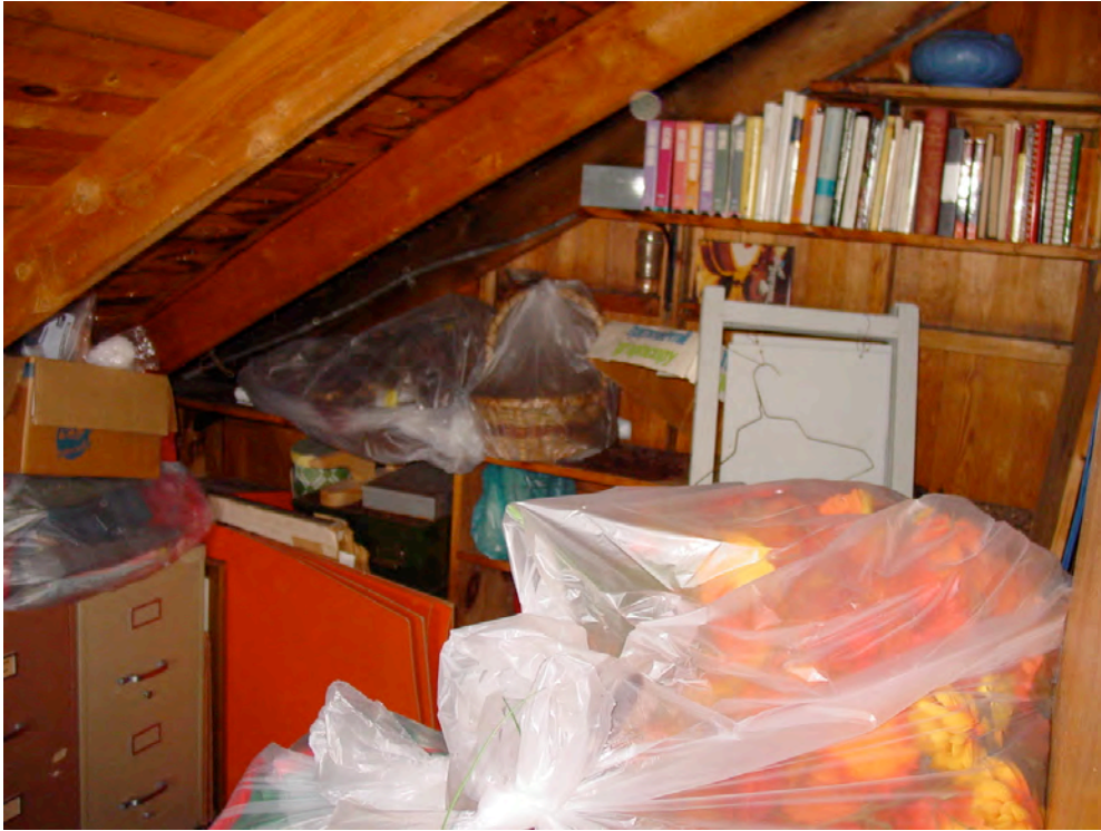
PR-3a: Storage area in southwest attic.
