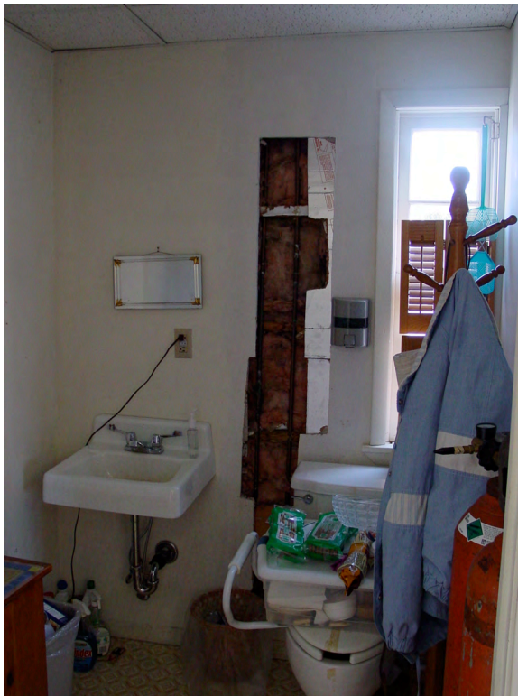
IC-4b: Handicapped accessible toilet room, unused.
