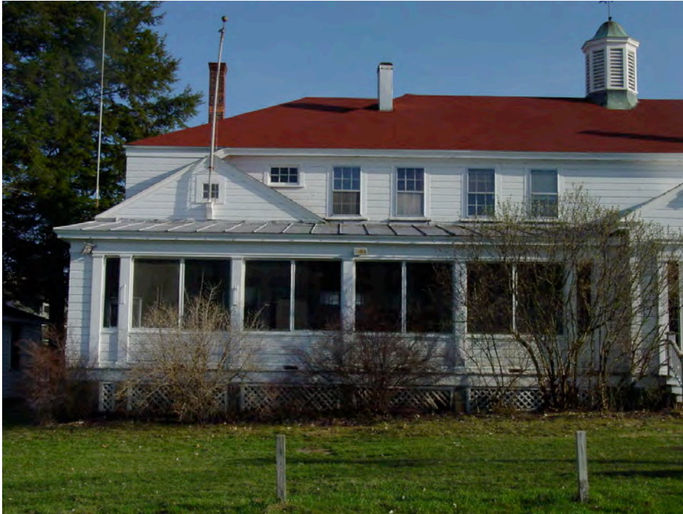
AI-1: The north or back porch, apparently a later addition.
