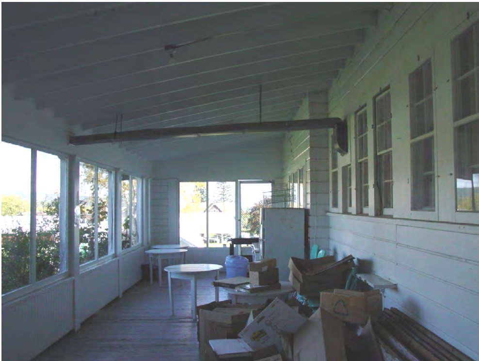
PR-2d: Back (north) porch, used for miscellaneous storage and for County Fair activities.
