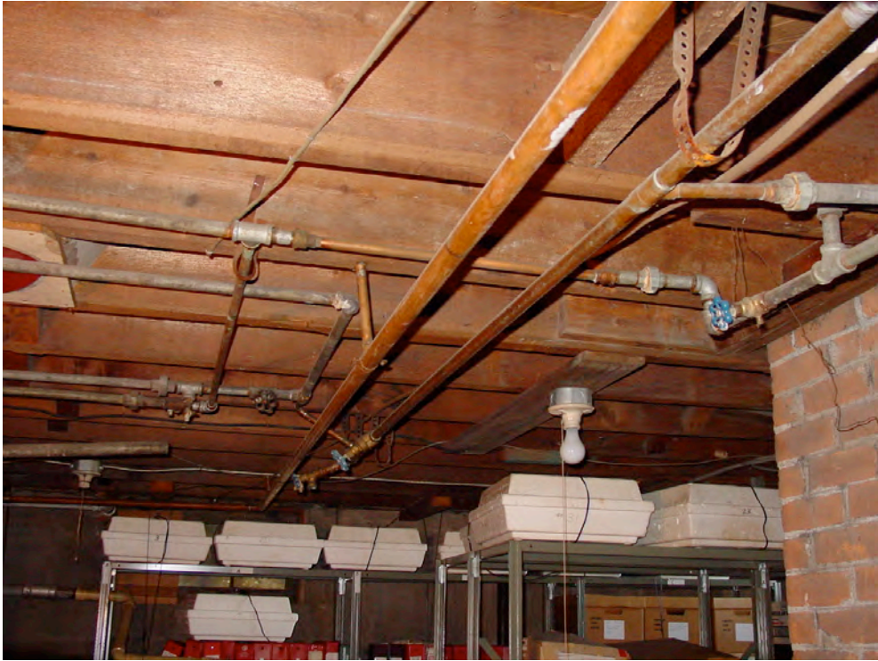
AI-7: Boiler room ceiling.
