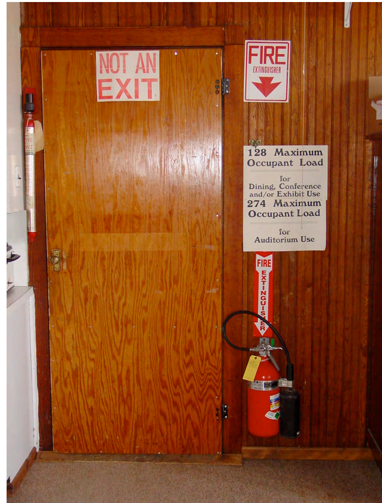
AI-4: Main assembly space with varnished bead board finish and five-panel door covered with plywood.
